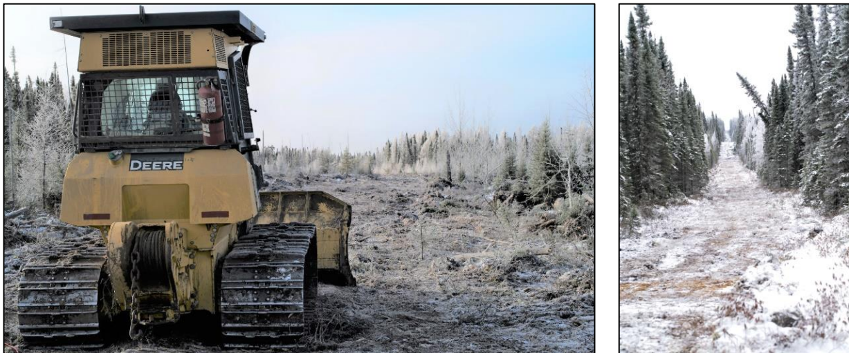
Figure 6-Progress on the Kasagiminnis Winter Access Track
